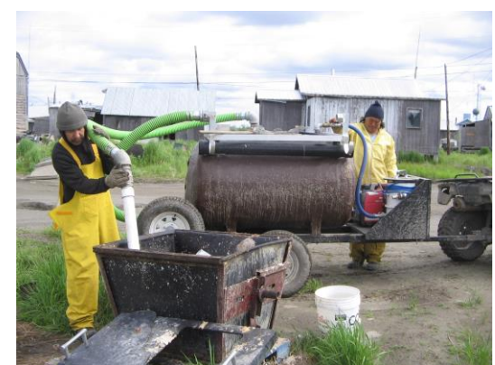
Using new tank, for safer transport of human waste.
