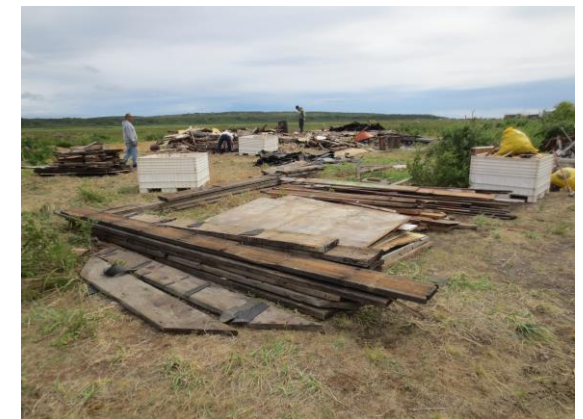
Dismantled lumber being staged for re-use
