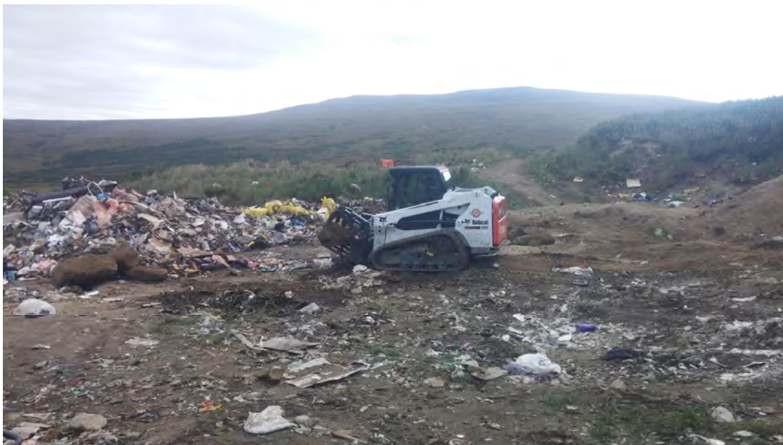
(To assist in keeping in the work face the grapple forks was used to move boulders)
