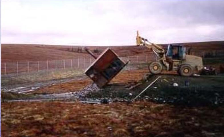
One of the bad things about burning-- You still need to deal with the ash. To empty the ash, people tilt this burnbox with a dozer. But burnboxes can be made with a handle to tilt by hand, or you can shovel the ash out.
