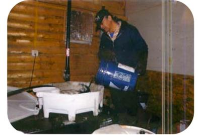
*Used oil is poured through a splash guard into the burner – which heats the tribal office.*
