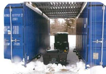
*Two connexes support a roof that shelters hazardous waste as well as program workers.*
