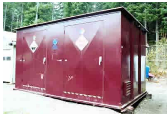
Glacier Bay National Park Landfill Hazardous Waste Storage Unit
