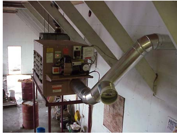
Installation complete! Note the chimney stack
