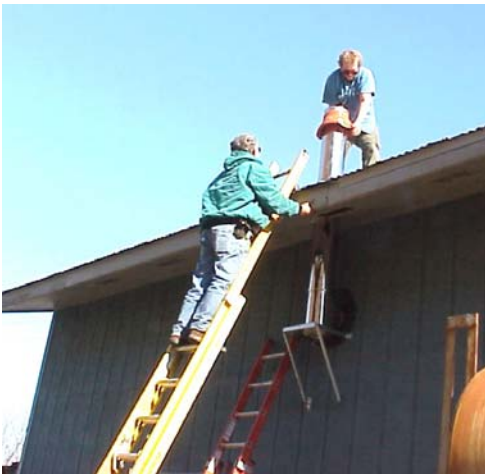
Feeding the stack from the inside of the building to the outside
