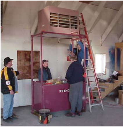
Installing the heater unit on top of the stand
