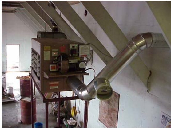
Feeding the stack from the inside of the building to the outside
