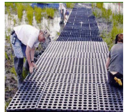
Photo Courtesy: Geochem, Inc.
