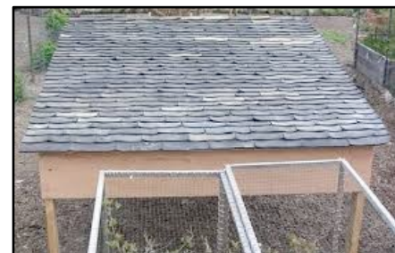
Waste tires used as roof shingles
